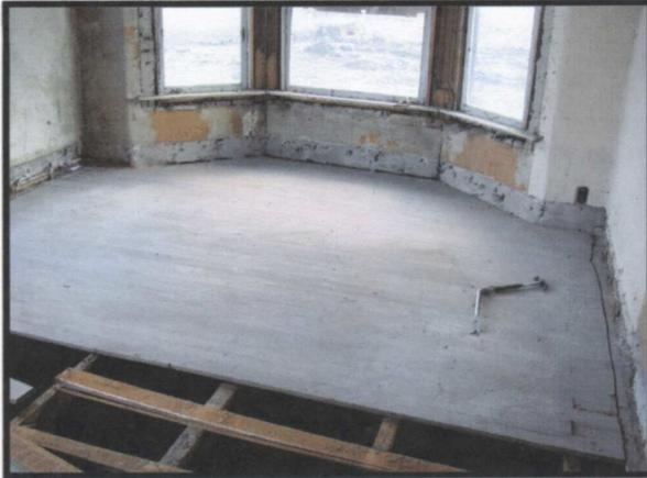
**This view is of the floor in one of the upstairs bedrooms. After so many decades of use the tongue and groove boards are in wonderful condition. Due to time constraints the easiest method for removal was to use a chain saw to cut an edge along the wall and then remove the boards one at a time.**
