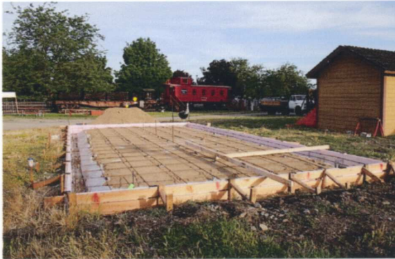
It's 7:00 in the morning on May 16. The forms and rebar are in place as we wait for the first Savage Redi-Mix truck to arrive. — Tony Johnson photo
