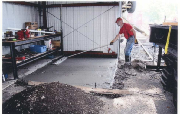
Jerry Hellinga estimated there would be less than one-half cubic yard of mix left so he had prepared forms inside the engine house for the excess. When it was filled there was less than a half wheelbarrow left. That's good figuring. — Tony Johnson photo
