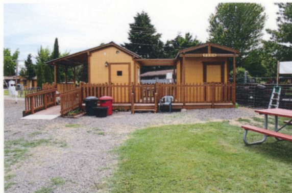
Our concession stand storage shed is finished. On June 2, Rick & Nancy Aubin finished applying the final paint. The buildings look good, don't they? Rick also surprised me by honoring my late father with his name on the shed. — Tony Johnson photo
