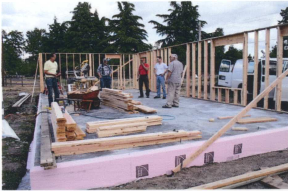
One week after pouring the foundation it was time to frame the walls. Larry Tuttle and Jerry Hellinga assembled the walls. Later on other members were called to help lift the walls in place. — Tony Johnson photo
