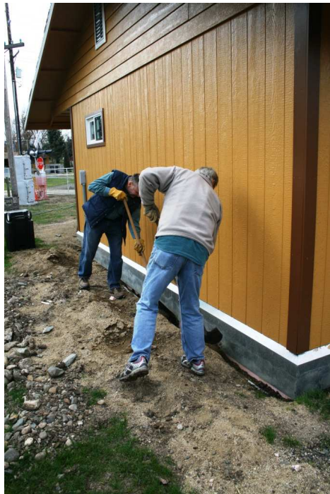
(ABOVE) This is the happy reaction of new member Walt May after learning he was volunteered to help us shovel concrete. (BELOW, and BELOW, RIGHT) Bruce McGarvey and Walt are busy shoveling fresh concrete to the required depth of two inches above the conduit. — Tony Johnson photos
