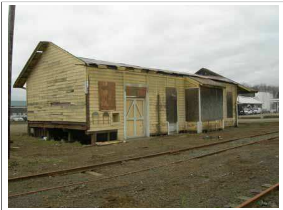
Roof and windows removed, the depot stood at its previous location, awaiting lifting and transportation
