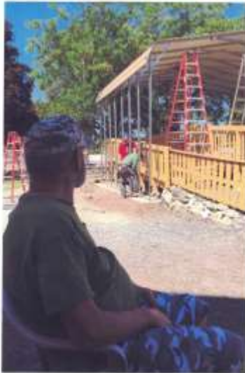
Ken is supervising the construction
